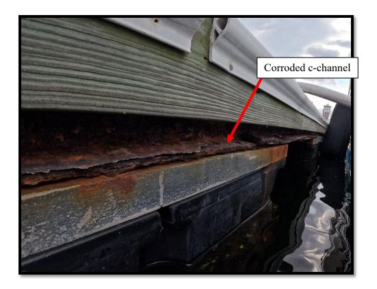
5) **Utility brackets** – Some of the utility lines are supported with metal brackets; many of the original brackets are rusted and or have been replaced due to corrosion.
