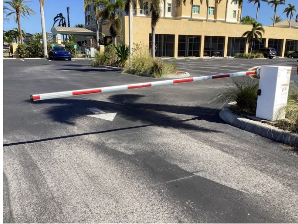
Typical gate operator with lift arm
