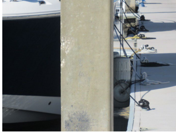
Minor concrete damage
