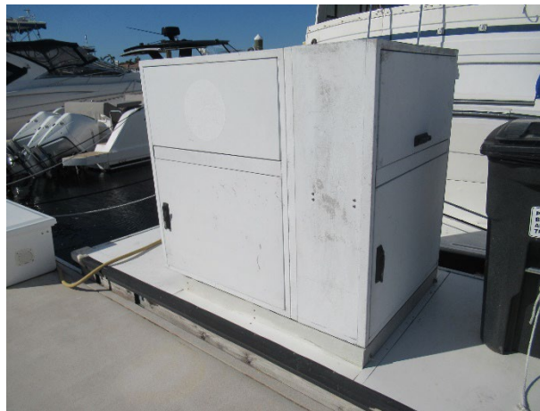
Typical electrical transformer, note discolored finishes
