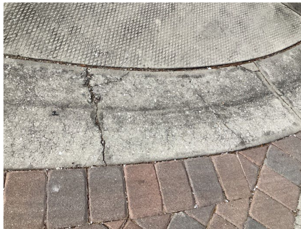
Concrete cracks
