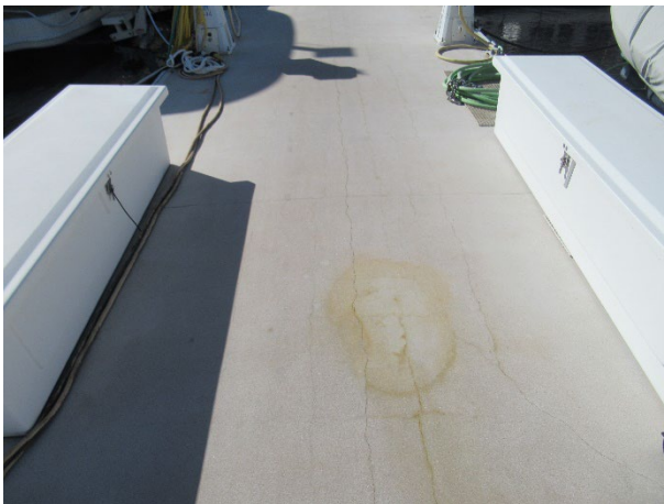
Dock surface cracks and staining
