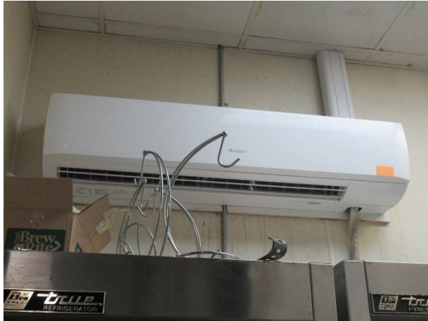
Newly added ductless mini-split system
