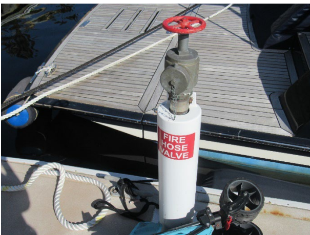
Typical fire protection standpipe
