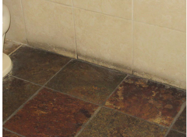
Discoloration and tile wear
