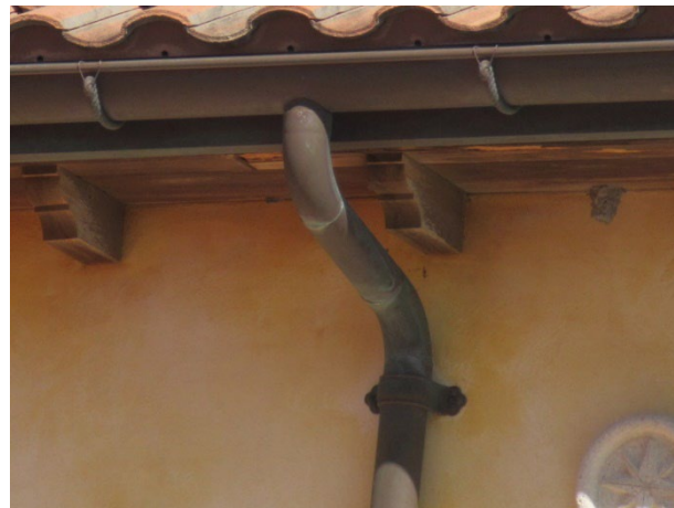
Evidence of leakage at seams and patina
