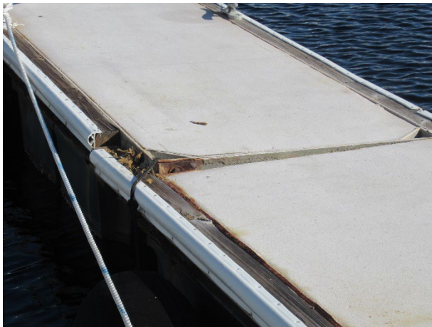
Damaged float assembly due to hurricane damage, note rust
