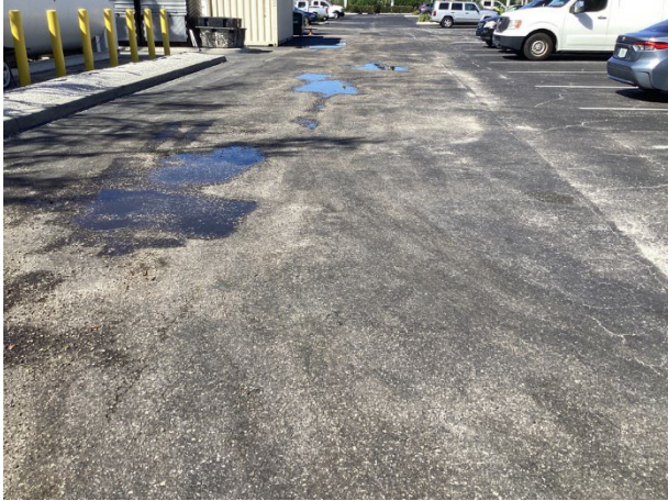
Phase 1 pavement overview, note patching and raveling
