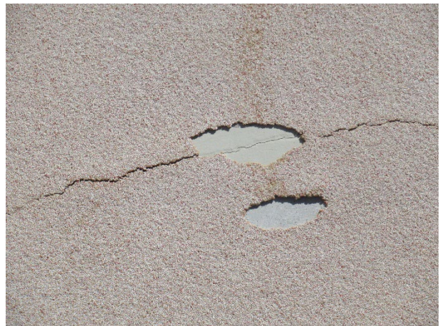
Coating cracks and missing coatings
