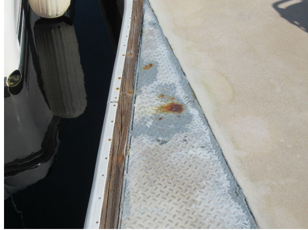
Corner gusset plate with rust
