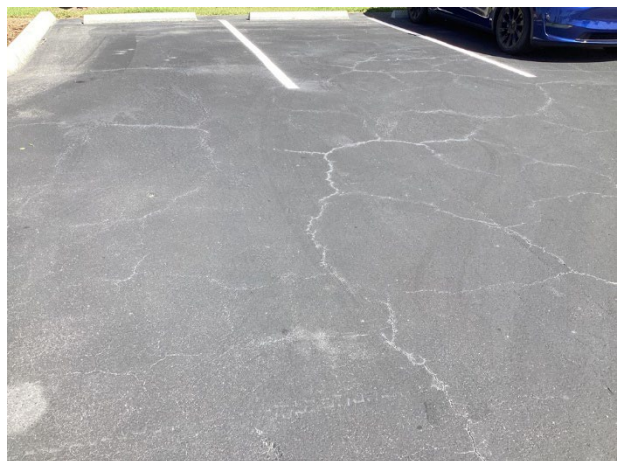
Phase 2 surface cracks
