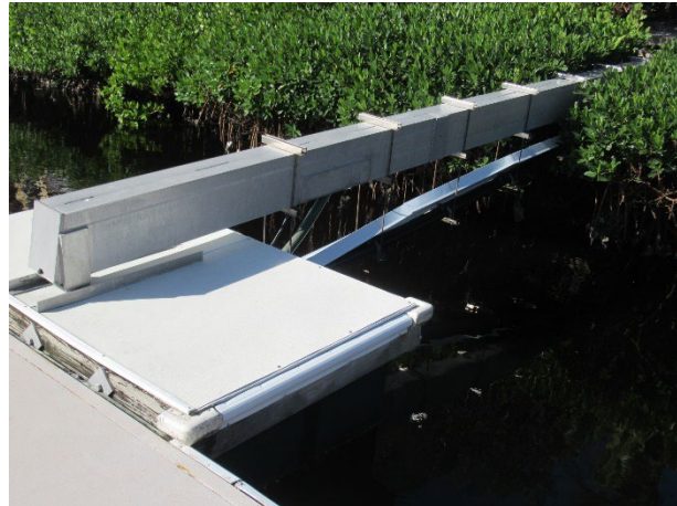
Fuel supply lines (cover to be reinstalled)
