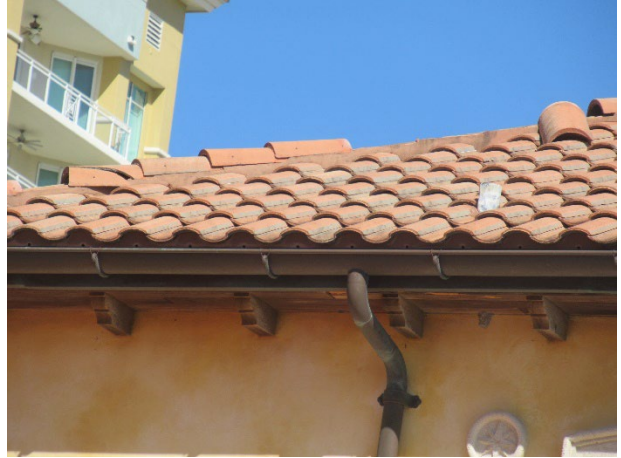
Missing and cracked tiles
