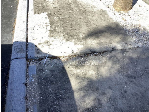
Heaving, potential trip hazard and damage along main walkway
