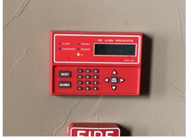
Annunciation panel to be replaced
