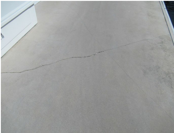
Significant crack at north dock
