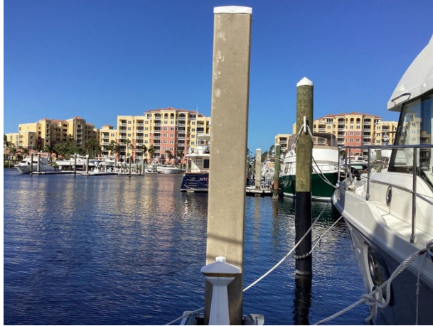
Concrete and wood pilings
