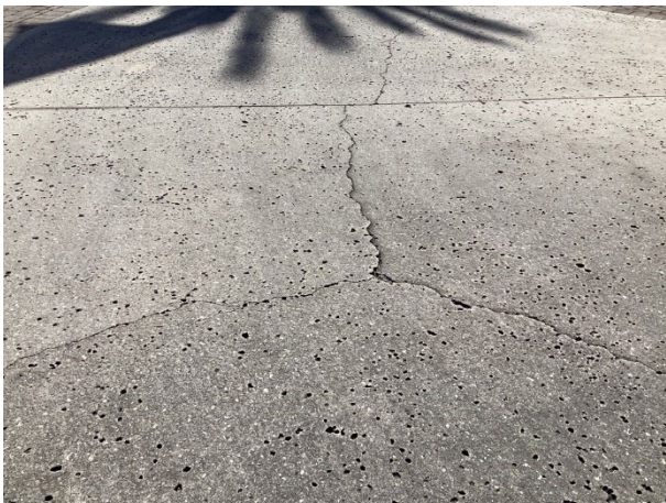
Concrete drive cracks
