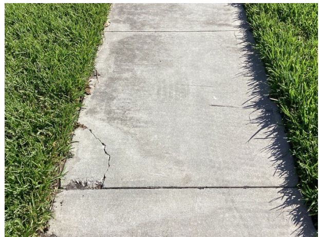
Isolated cracks and damage
