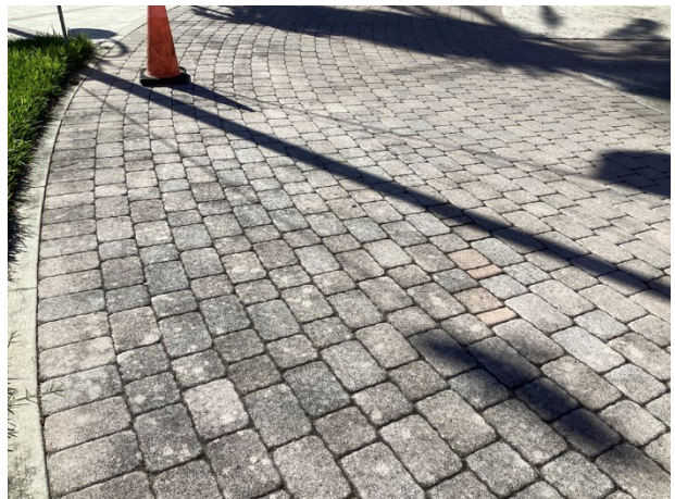
Vehicular paver deterioration and staining
