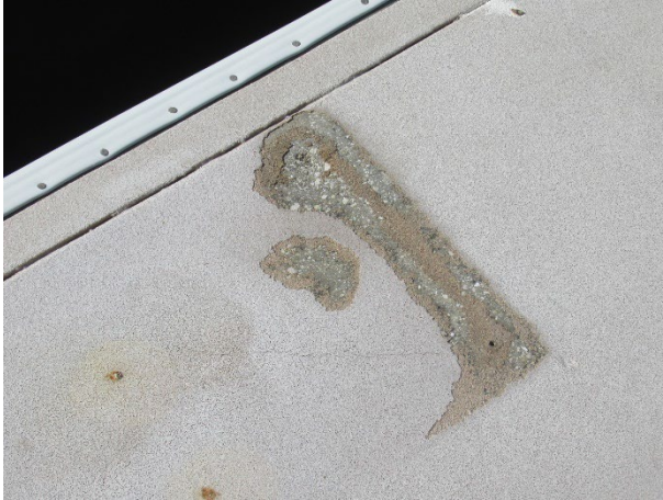
Surface damage at removed dock box
