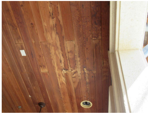
Wood soffit below, note evidence of water infiltration
