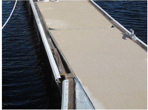
Damaged float assembly due to hurricane damage
