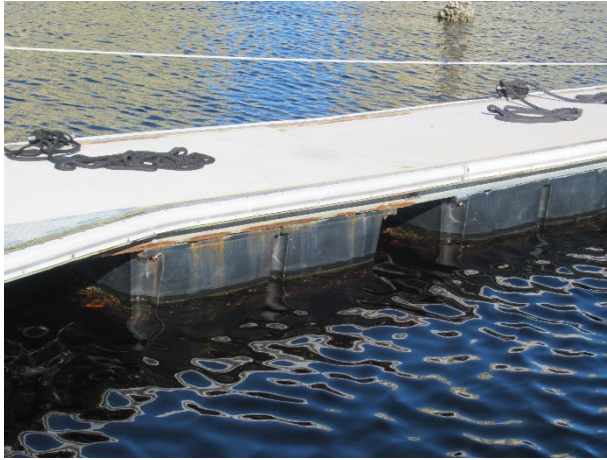
Float assembly with rust
