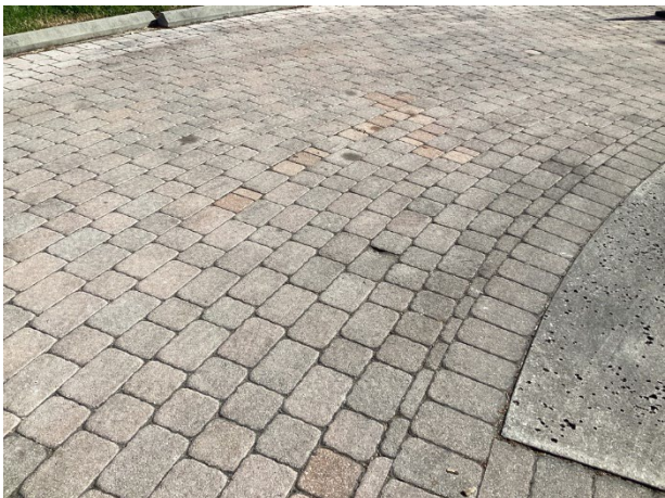
Vehicular paver deterioration, settlement and limited replacements
