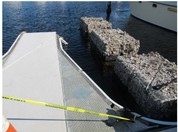
Overturned float due to hurricane damage
