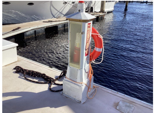
Typical fire extinguisher pedestal
