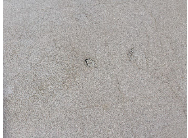
Coating cracks, deterioration and missing areas
