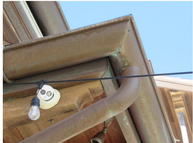
Evidence of leakage at seams and patina
