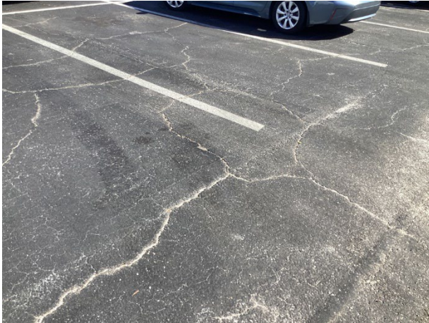
Pavement cracks at Phase 1
