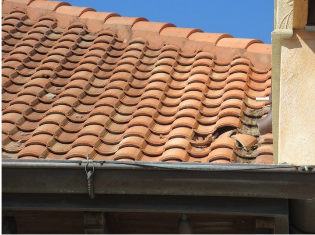
Area of damaged tiles
