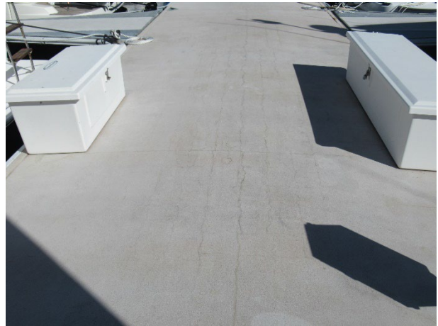
Dock surface cracks
