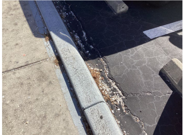
Pavement edge cracks, note sidewalk settlement along curb
