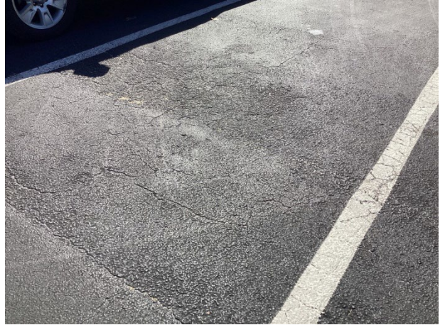
Pavement surface cracks and deterioration
