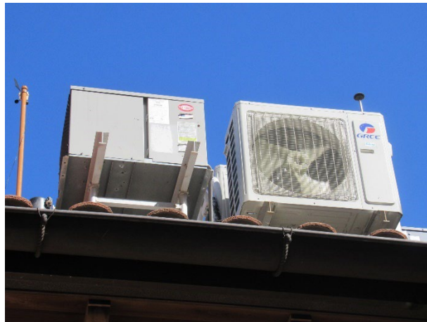
Walk-in condensing unit (left) and mini-split condensing unit (right)
