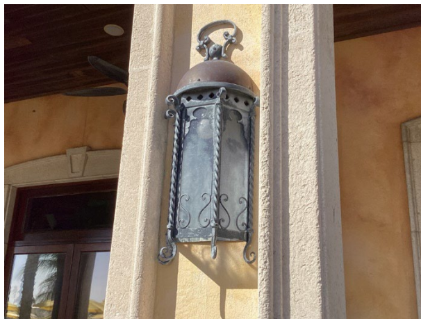
Wall mounted light fixture, note weathered finishes
