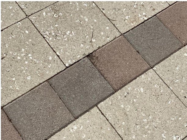
Minor paver deterioration
