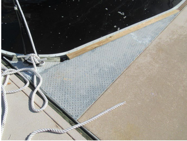
Replaced corner gusset plate
