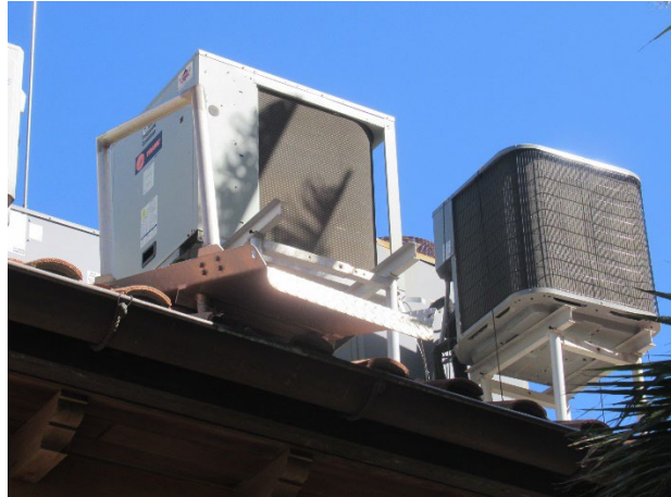
Split system condensing units
