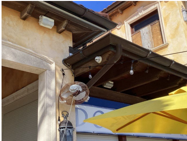
Copper gutters and downspout
