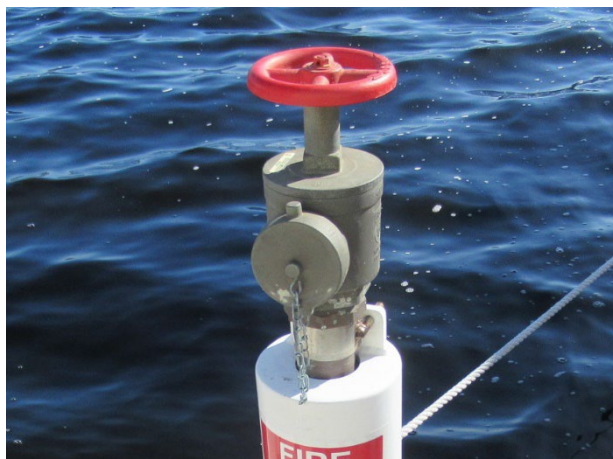
Fire protection standpipe, note corrosion onset
